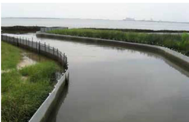
Figure 5. Adsorbent fabric fences prevent oil from crossing the barrier but water can pass through for drainage.
